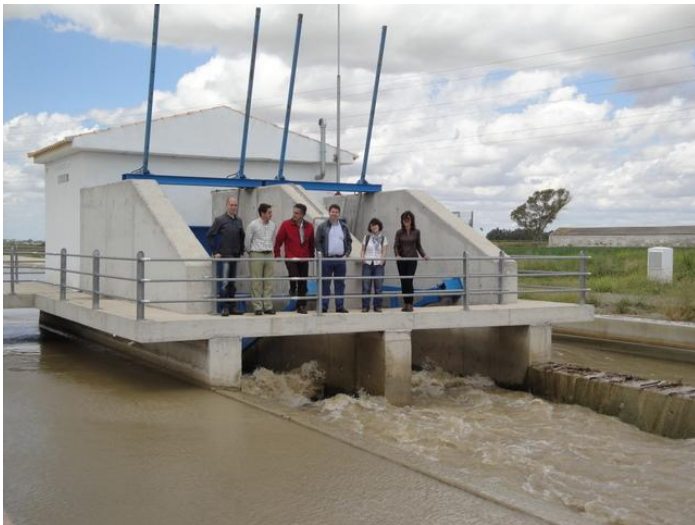
Two Taintor Gates with side weirs
